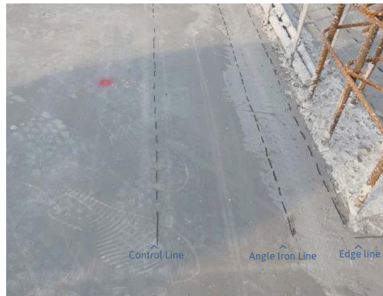
Control line, Angle Iron line, Edge line
